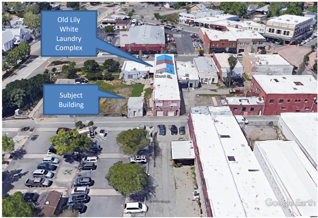
Figure 9: Aerial Photograph of the project site and subject building (Google Earth 2018).
